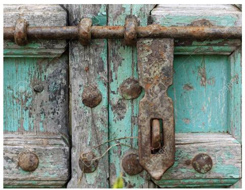
The cypress wood has a distinct, somewhat sour odor while being worked, rated as being durable to very durable in regards to decay resistance. The years and the elements haven't been kind to the exterior of this 94-year-old, thick, cypress door - said the carpenter. Flakes of varnish still clung to the wood in spots, while the rest of the surface was rough and dried out from the effects of water and sun. Well, it could take a long to restore it - he added – but it was worth it.
